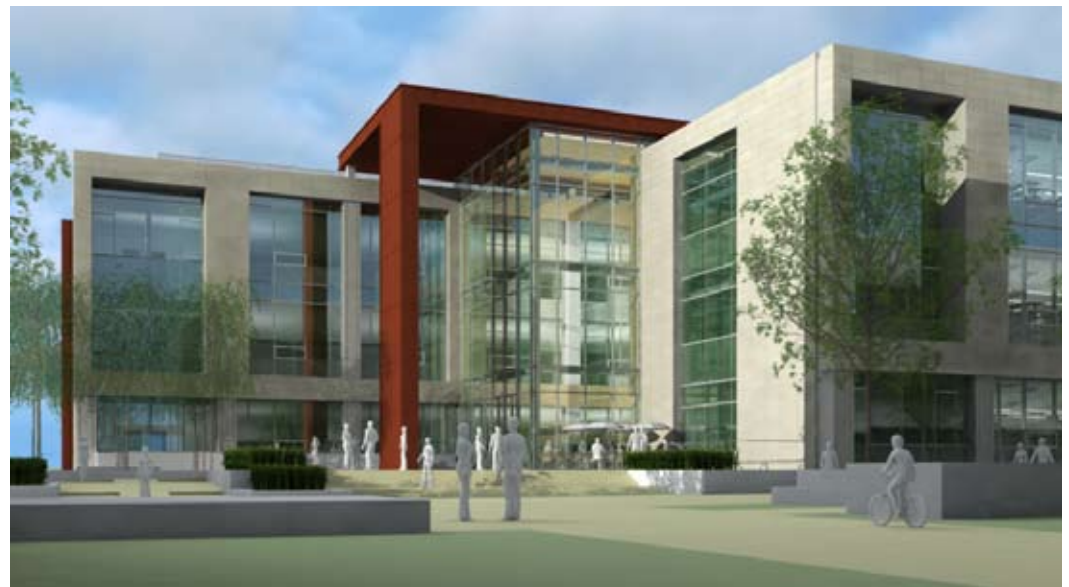
Entrance to the northeast corner of the building
