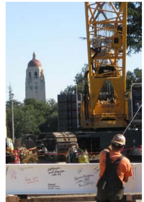
The last piece of steel lifted into place
